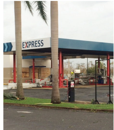
Hurricane Maria damaged Fort Buchanan’s Express.
