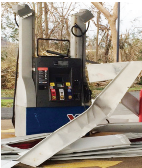
The Express at Fort Buchanan was damaged by Hurricane Maria.
