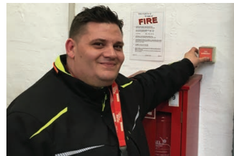
Germersheim DC's Christian Nord checks automated fire doors that separate his warehouse from an adjacent one.
