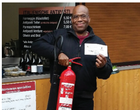
During the holidays at KMCC, Services’ Frank Hines confirms that Christmas Market huts have extinguishers.
